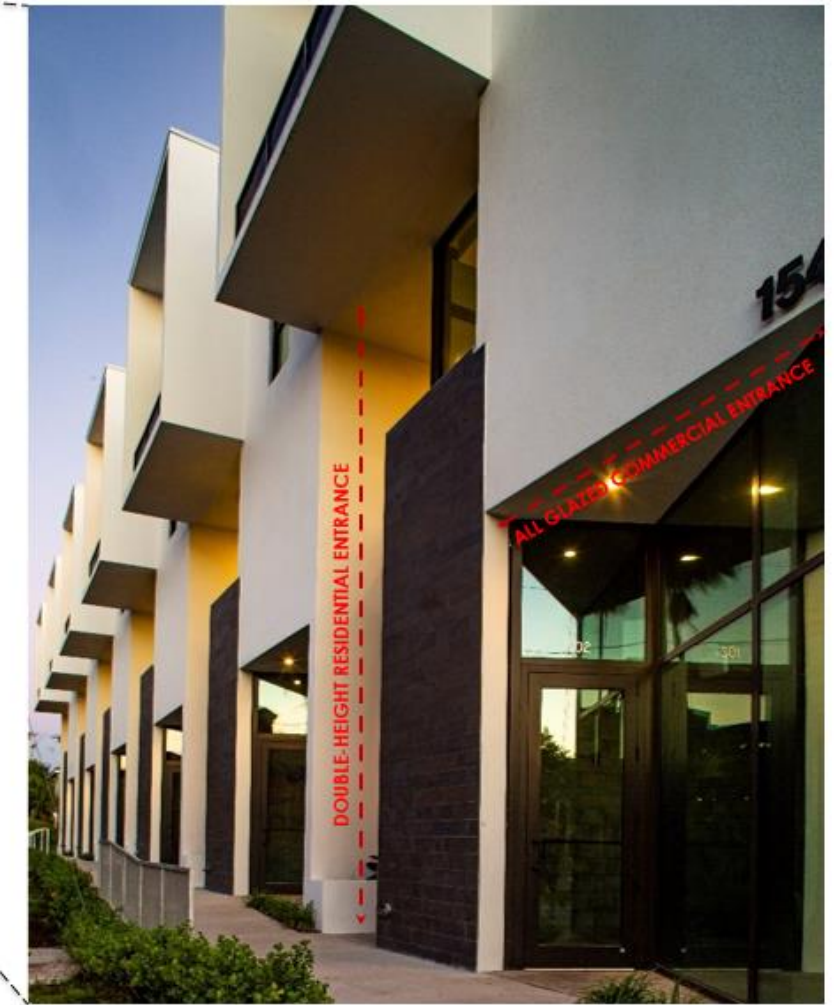
THE RESIDENTIAL AND COMMERCIAL ENTRANCES CONTRAST WITH ONE ANOTHER. ONE IS VERTICAL AND PRIVATE; THE OTHER IS ANGLED AND TRANSPARENT ADDING TO THE RHYTHM OF THE STREET.
